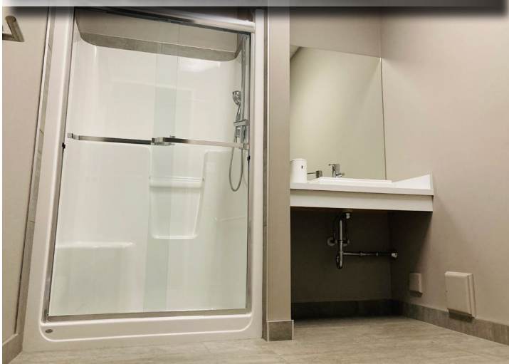
MAIN FLOOR WASHROOM WITH SHOWER
