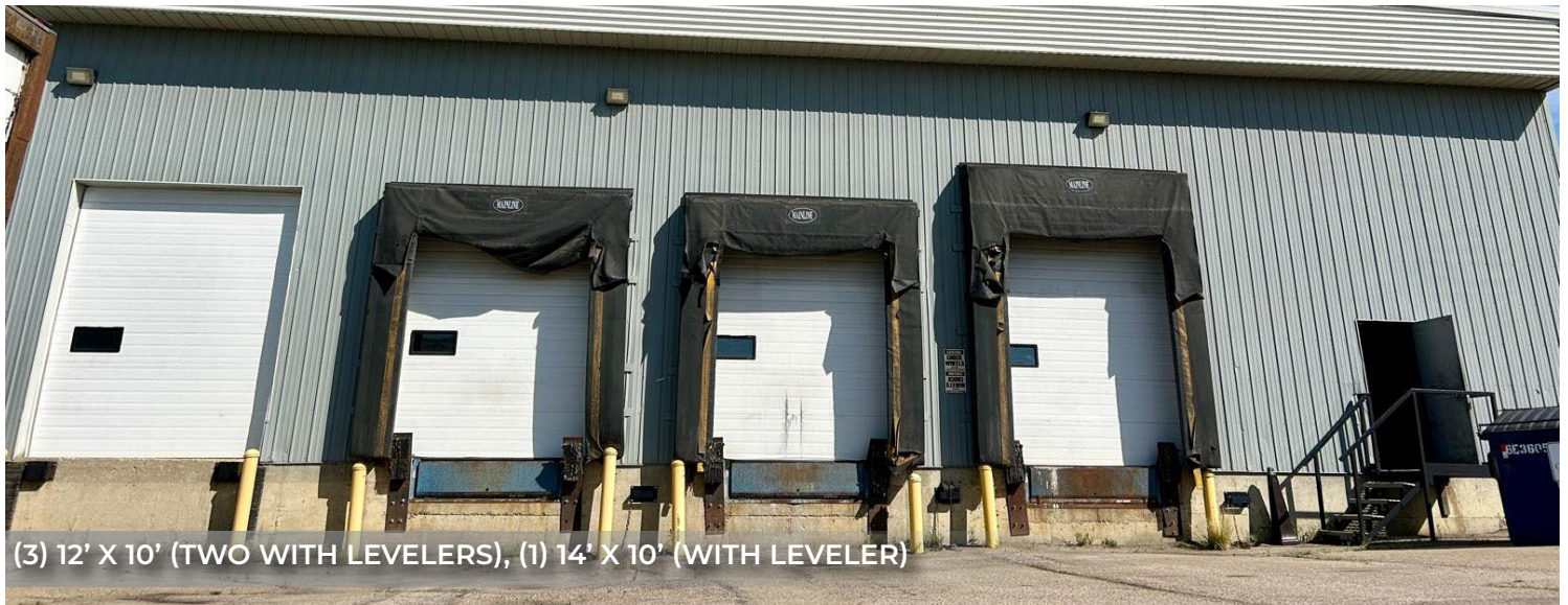
PAVED MARSHALLING AREA WITH DOCK LEVEL LOADING DOORS, BUMPERS, AND LEVELERS
